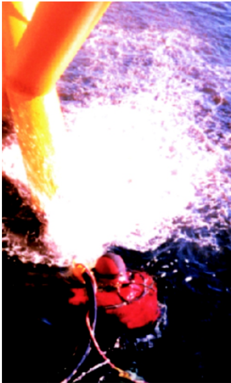
Top left: A diver prepares the surface for coating using grit-blasting equipment. Top right: The coating is applied by hand brush straight from the tin. First, an index coating of black followed by a top coat tinted to match the original polyurethane. Bottom left: The finished repair is indistinguishable from the rest of the structure. Bottom right: Underwater, the leg can be seen to be fully coated and protected.
