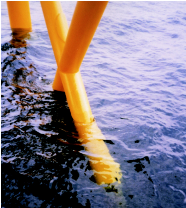
Top left: A diver prepares the surface for coating using grit-blasting equipment. Top right: The coating is applied by hand brush straight from the tin. First, an index coating of black followed by a top coat tinted to match the original polyurethane. Bottom left: The finished repair is indistinguishable from the rest of the structure. Bottom right: Underwater, the leg can be seen to be fully coated and protected.
