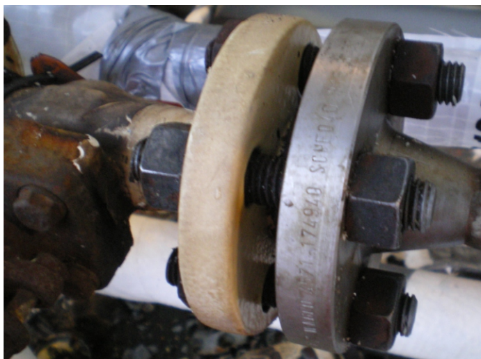
Fig 4: a mixed stainless and carbon steel joint with carbon steel bolts with Enviropeel encapsulation removed after more than 6 years
