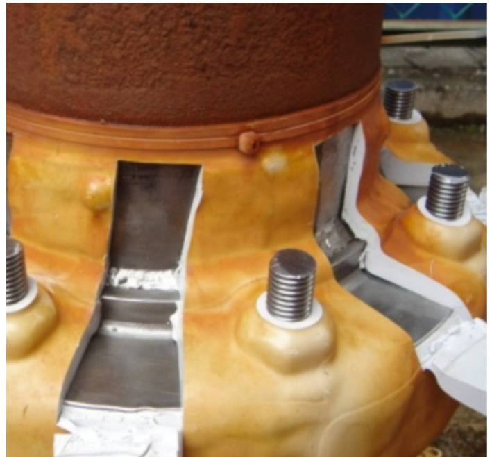
Fig 8 below: initially, strips of Enviropeel are removed from the substrate.
