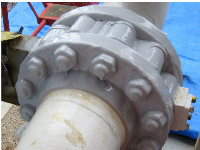
Fig 4: a mixed stainless and carbon steel joint with carbon steel bolts with Enviropeel encapsulation removed after more than 6 years
