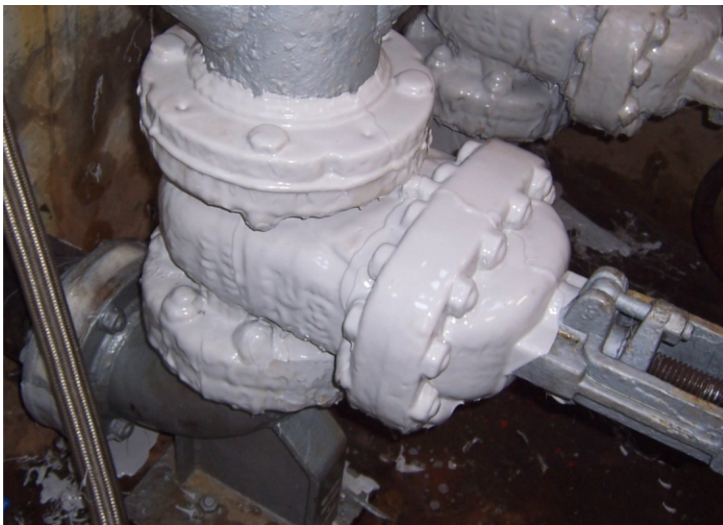
Before and after of encapsulation using Enviropeel 170.
