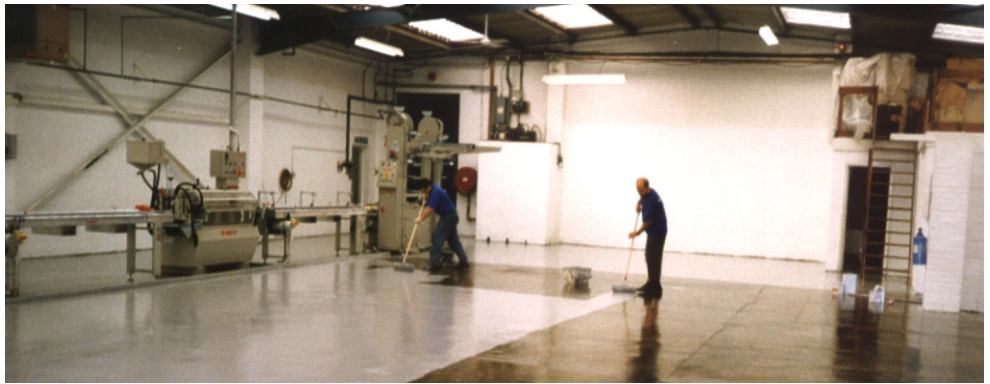
The pictures show, from the left, stripe coating the edges, application of 28.95 then 28.15 by roller and, finally, the finished floor.
